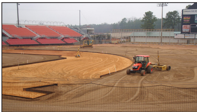
Laser Grading a Baseball Field – Photo courtesy of Brad Fresenburg, Ph.D.
