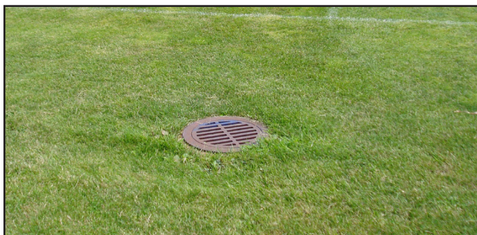
Exposed objects, such as this drain, can create safety hazards for athletes. Photo courtesy of Pamela Sherratt.
