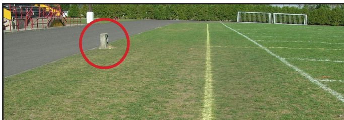
The concrete box in the out of bounds area should be properly padded to protect athletes. Photo courtesy of Pamela Sherratt.
