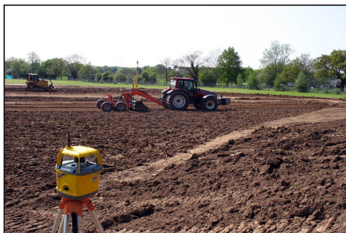
Laser Grading – Photo courtesy of Brad Fresenburg, Ph.D.
