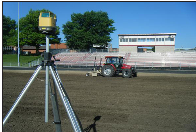
Laser grading a football/soccer field – Photo courtesy of Brad Fresenburg, Ph.D.
