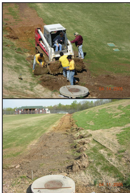
Example of bad conduit installation along edge of a natural turfgrass field and reconstruction to fix it. Photo: Tony L. Strickland, CSFM
