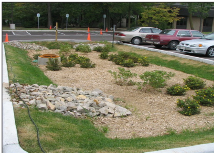
Bioretention area/rain garden utilizing native plantings - Picture courtesy of Aaron Volkening, P.E.
