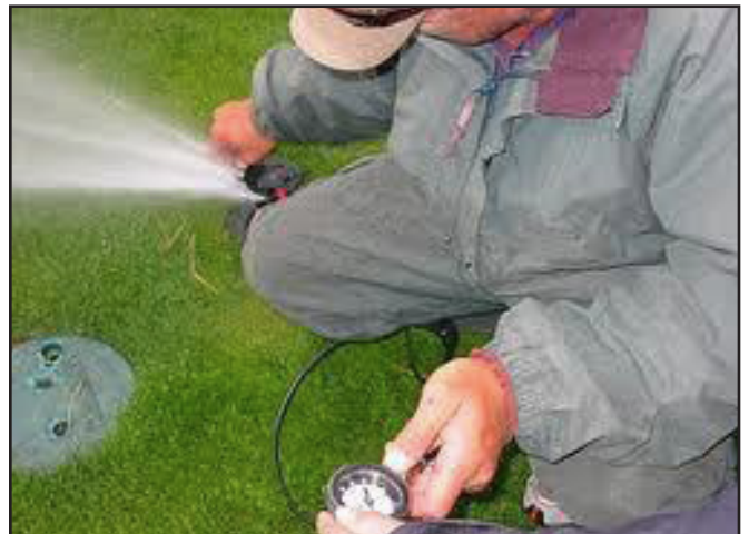
Measure operating pressure – Photo courtesy of Jeff Gilbert
