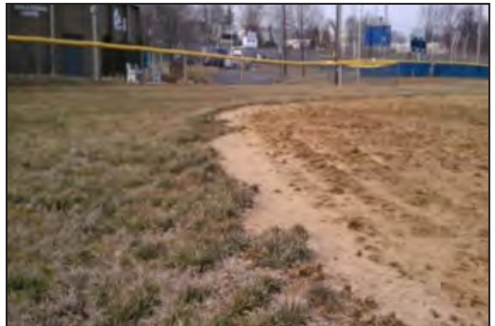
A 12-inch elevation change (lip) between the infield skin and outfield. The transition from infield to turfgrass should be flat. Photo courtesy of Scott Bills, CSFM.
