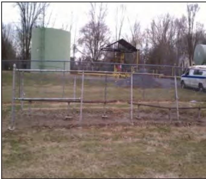
Unstable benches and exposed concrete footings in team areas present a safety hazard. Photo courtesy of Scott Bills, CSFM.
