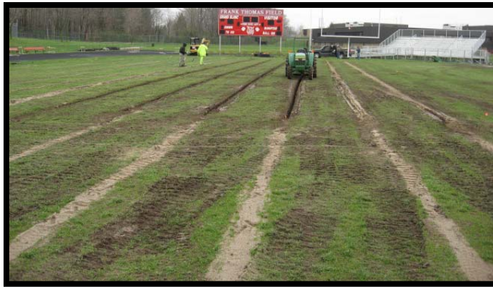
Image 1: Cutting drain lines, installing drain tiles, and backfilling lines with a sand-based root zone material, Grand Blanc High School, Grand Blanc, Mich., Water Management Inc., May 2007.
