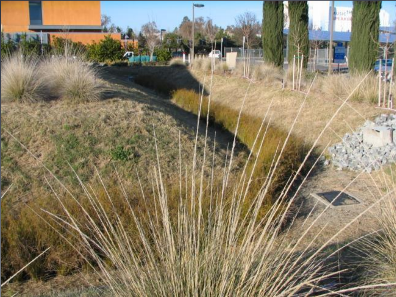
Storm water detention basin
